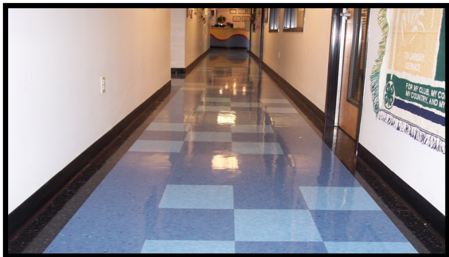
Fort MacArthur, San Pedro, CA Youth Center: Replaced VCT Tile Floor and Cove Base; Repaired/Replaced Subfloor; Painted Interior Walls Call Henry, Inc. - Jose Perez (310) 597-3323
