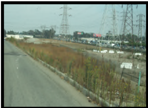
Air Force Lot, Pico Rivera Cleared 13 Acres (i.e., Weeds, Brush, Trees, Trash, Concrete, Asphalt, Gravel, Mobile Homes, Etc.); Sprayed Weed Killer & Pre-Emergent; Planted 13 California Native Trees (24" box) Call Henry, Inc. - Jose Perez (310) 597-3323
