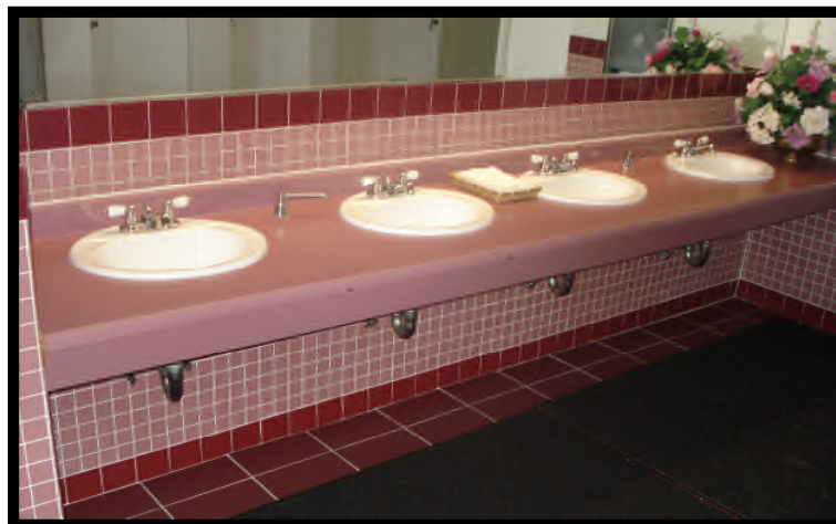
Fort MacArthur, Pacific Crest & Pacific Heights, San Pedro, CA Bldg. 403: Replaced Tile and Subfloor in Men's Restroom Call Henry, Inc. - Jose Perez (310) 597-3323
