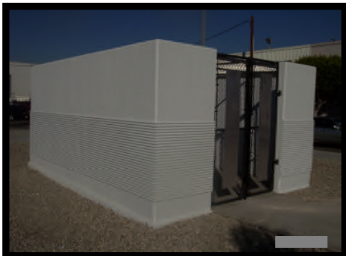
Los Angeles Air Force Base, El Segundo, CA Bldg. 281: Constructed Trash Enclosure With Concrete Pour-In-Place Walls, Foundation Call Henry, Inc. - Jose Perez (310) 597-3323
