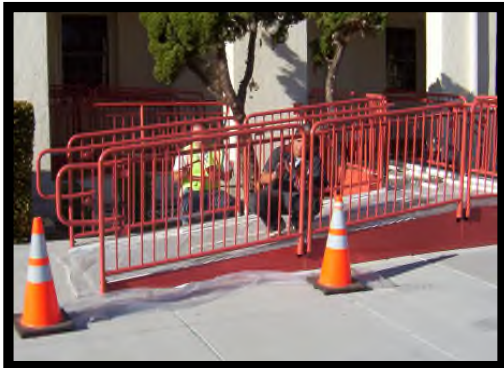
Fort MacArthur, San Pedro, CA Installed Handicap Ramps & Handrails; Converted Manual Doors to Automatic Call Henry, Inc. - Jose Perez (310) 597-3323
